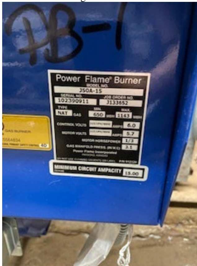
Photo of Existing Power Burner Data Plate
